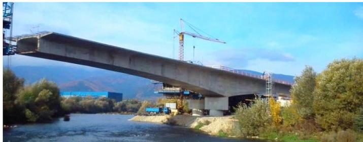
Figure 1. Bridge No.205 - left cantilever V1 – the final construction stage.
